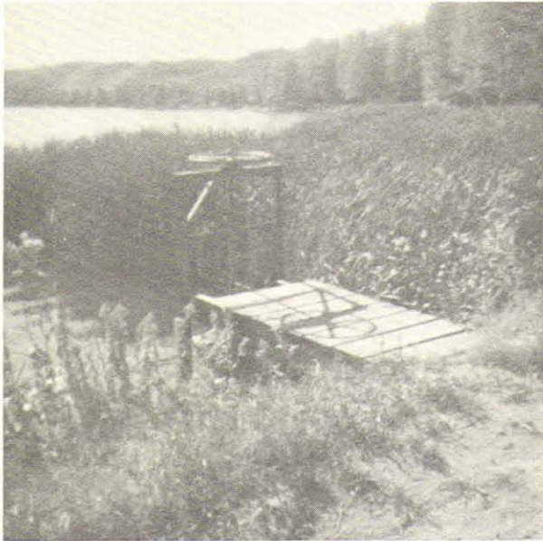
Dam gate that is holding water back from cattle.
